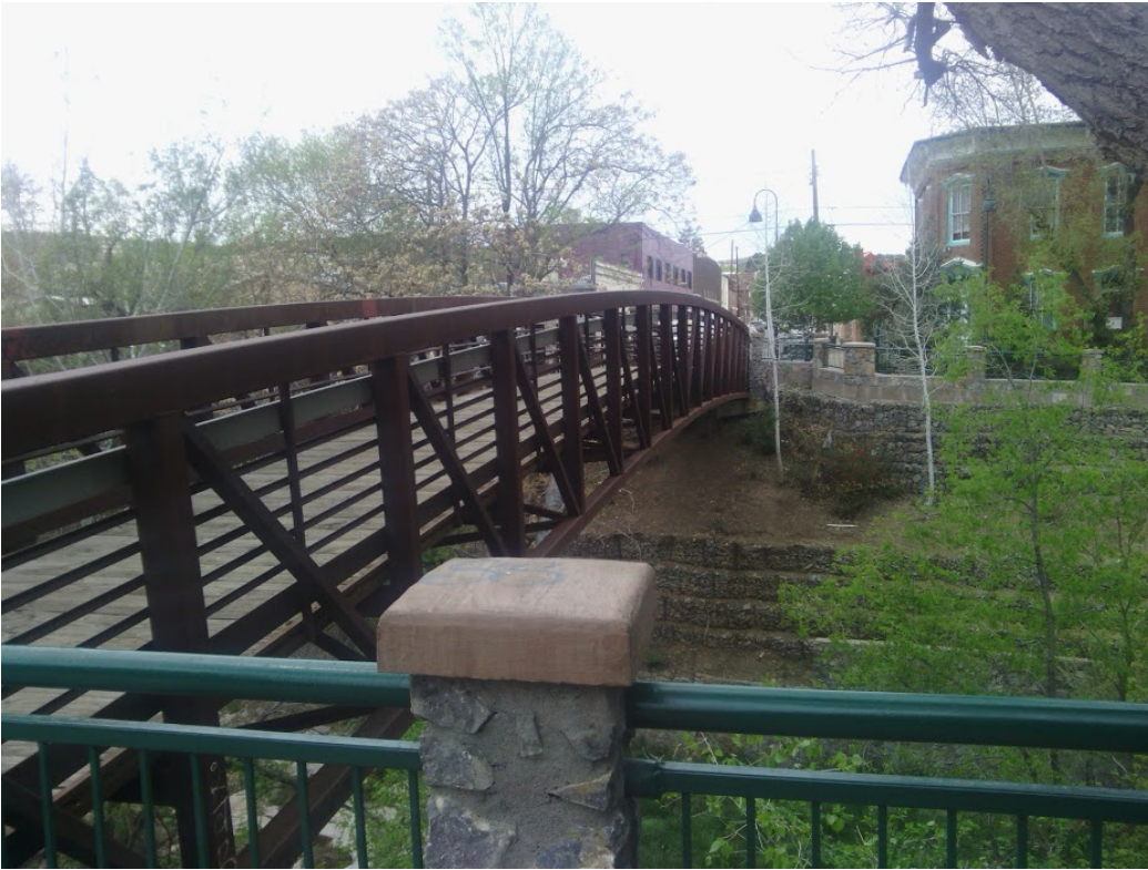
Pedestrian bridge across "big ditch" in Silver City
