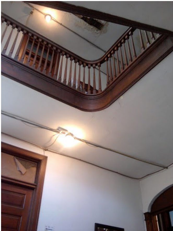
Tour of The Doyle rooms
