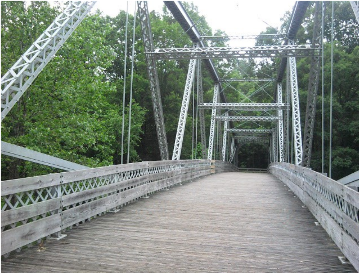
Swatara Creek footbridge
