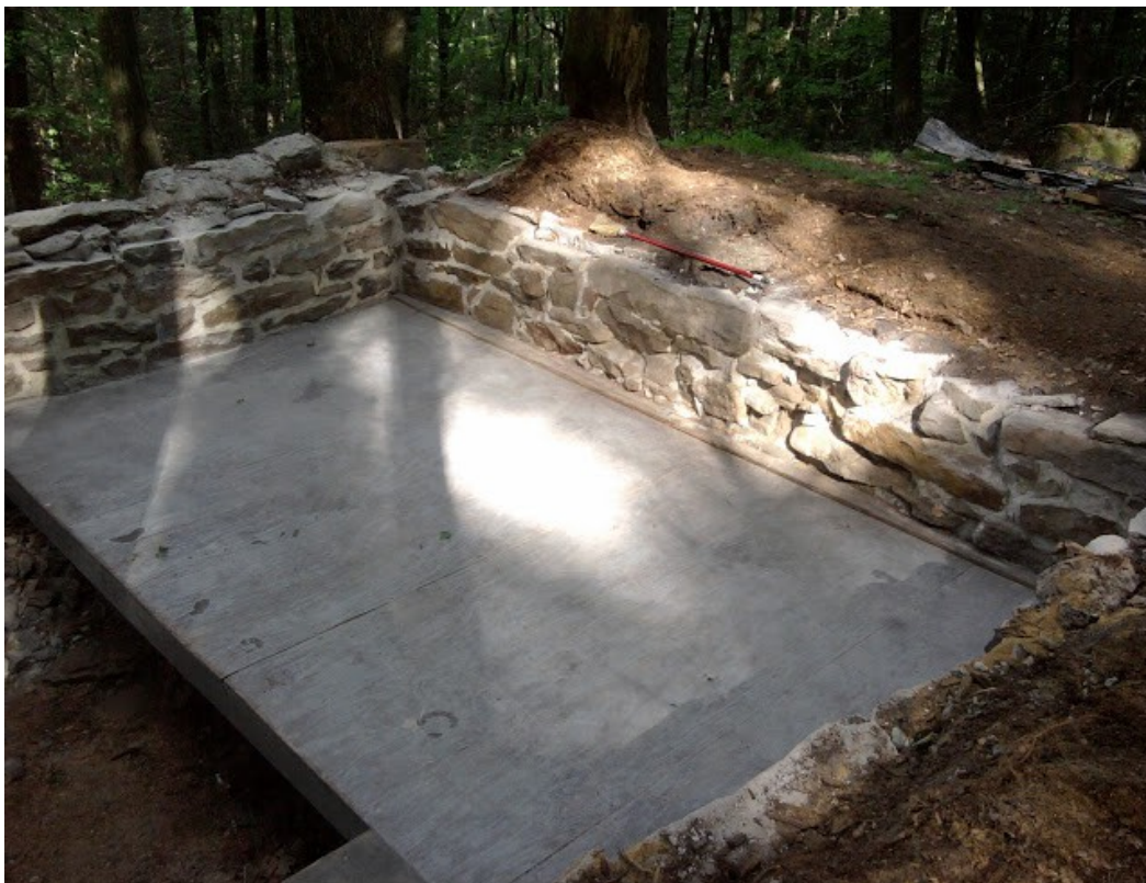
Rausch Shelter being reconstructed
