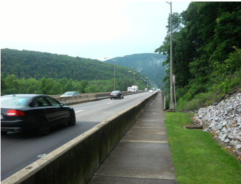
Delaware River Bridge
