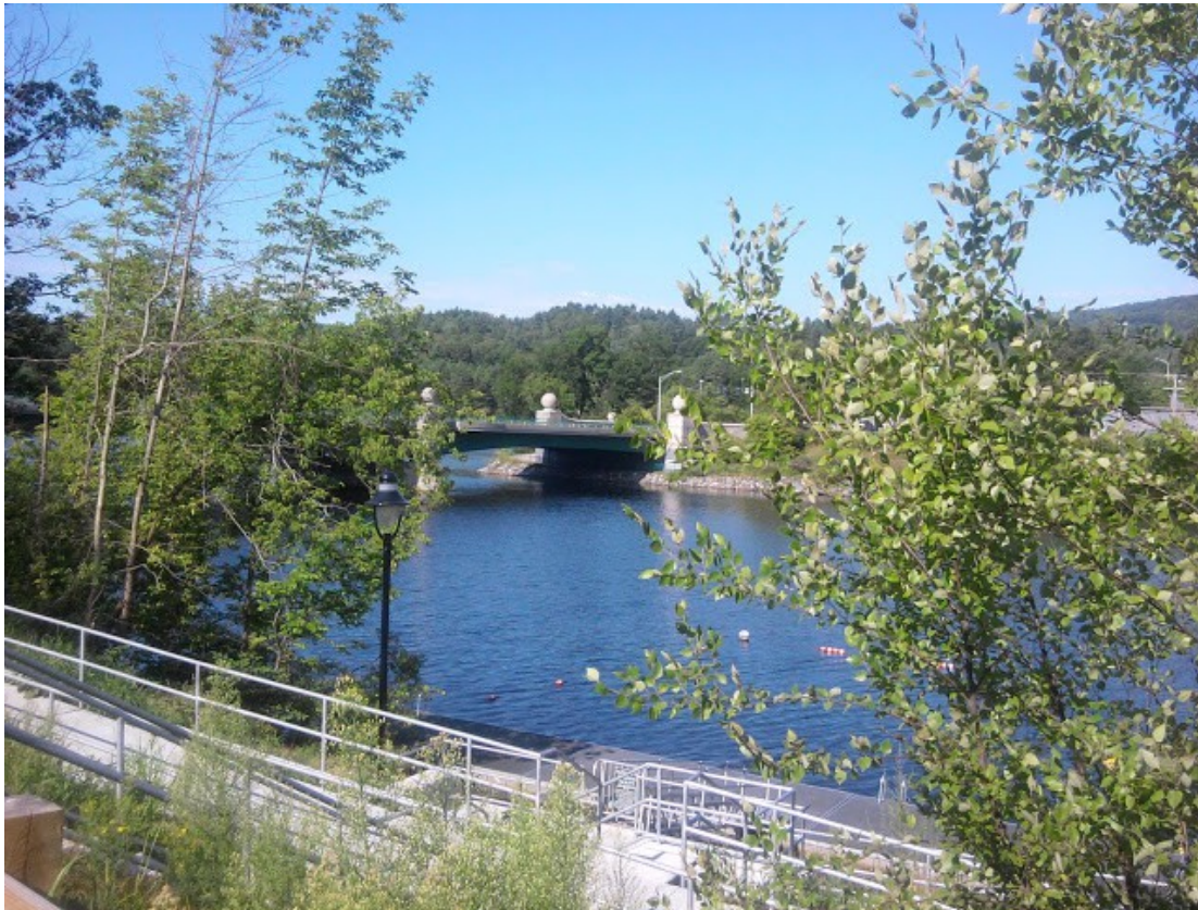
Bridge over Connecticut River, viewed from NH side
